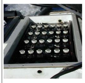
compensated. Hydrogen is captured on the top of each cover of tank. Safety valves open by themselves when hydrogen pressure is above 100mbar.
